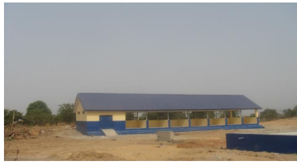
Kogi VCDP completed market stall at Kungbani, Lokoja LGA
