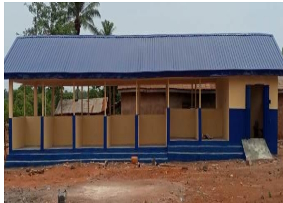
Kogi VCDP completed Market Stall at Imane, Olamaboro LGA
