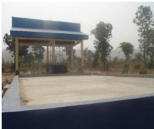
Kogi VCDP completed Parboiling shed and drying slab at Kungbani, Lokoja LGA
