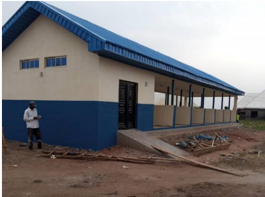
Kogi VCDP completed Market Stall at Egah Market Ibadan, LGA
