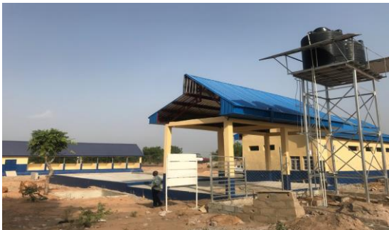
Rice Processors Centre, Market stall and a solar powered bore hole at kungbani, Lokoja LGA
