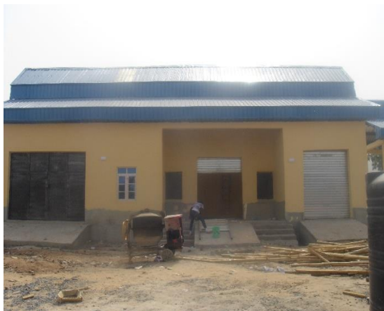
Kogi VCDP completed Rice Processing Mill at Kungbani, Lokoja LGA
